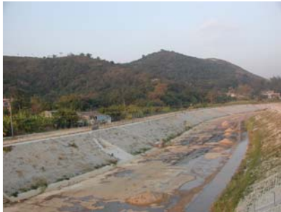
Ng Tung River, Fanling, after Channelization works
